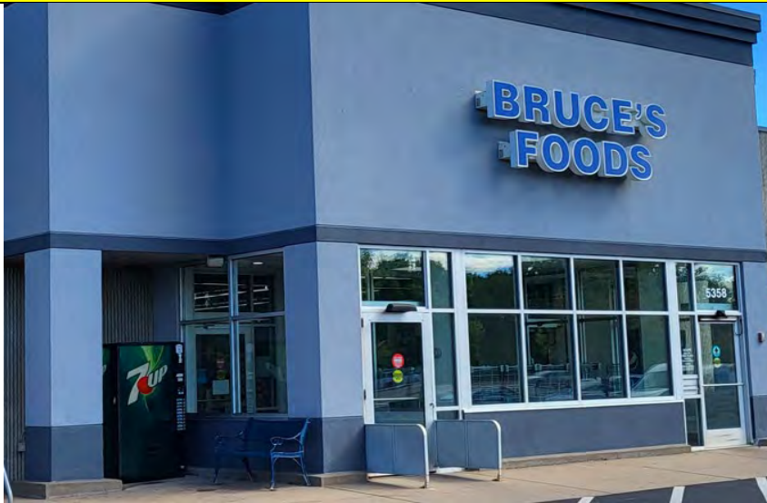
i Exterior finish installation system (EIFS) Bruce's Foods
