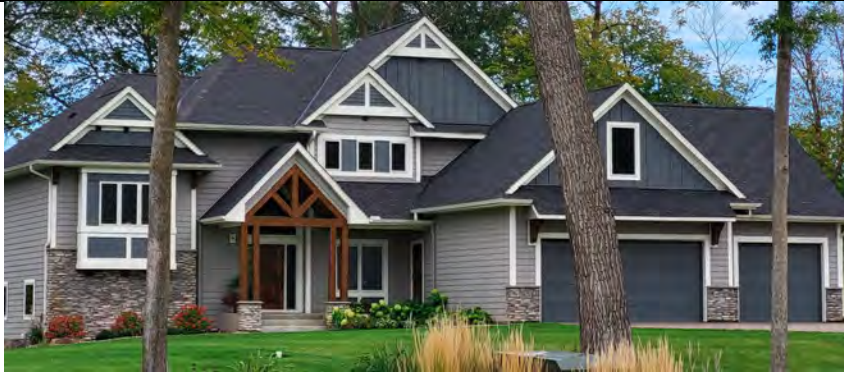
iv Fiber-cement exterior siding Home on West Comfort Drive
