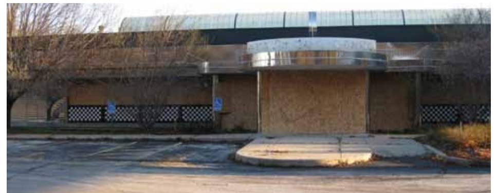
The vacant hotel and diner create an eyesore and nuisance problem today, but represent a strong redevelopment opportunity.
