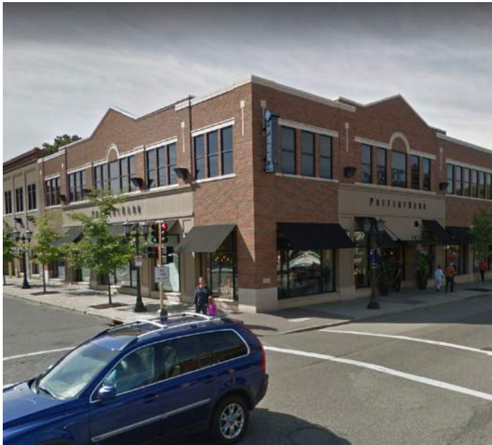
Public parking integrated with development (street view) example.
