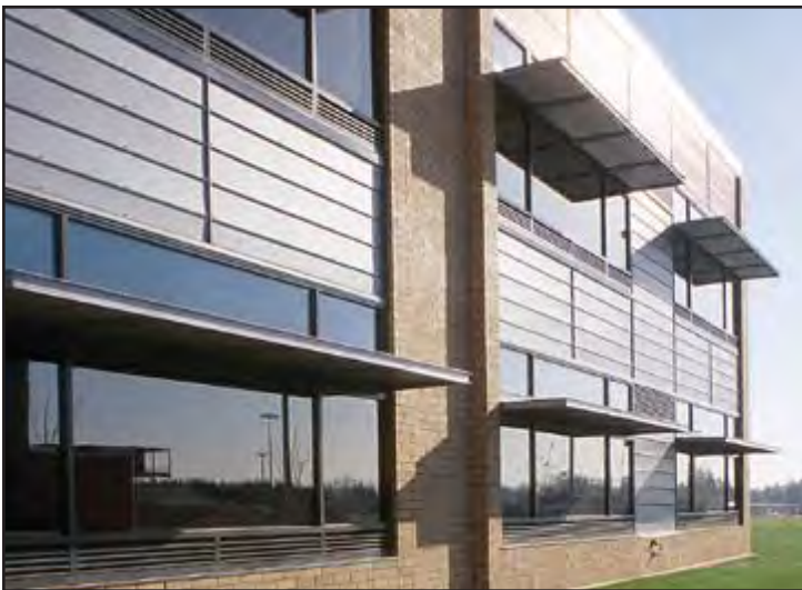
Sun Screens for Building Efficiency
