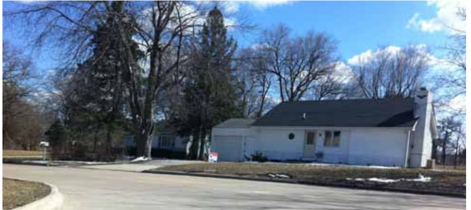
A handful of single family homes remain on the northern portion of the Heard Gardens site.
