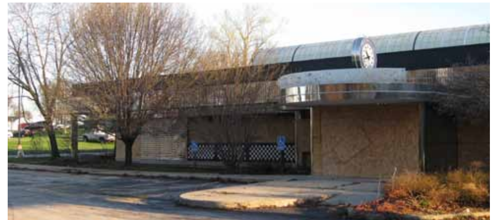
The former hotel and diner building need to be demolished to create redevelopment interest in the corridor.
