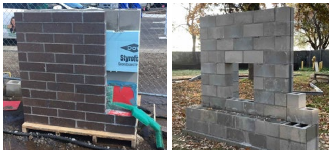
▲ Example pre-installation masonry mock-ups
