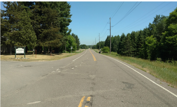
At Birchwood Terrace Looking North
