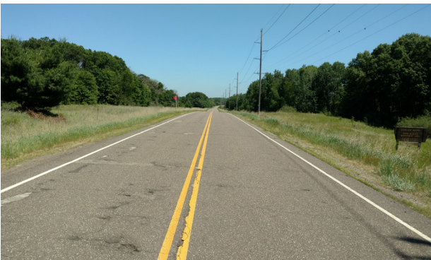
North of Birchwood Terrace Looking North
