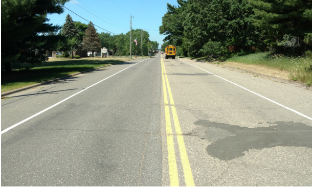
At Garden Lane Looking West
