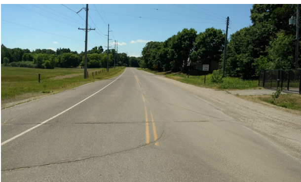
Railroad Boulevard (Transfer Station and Recycling Center) Looking South
