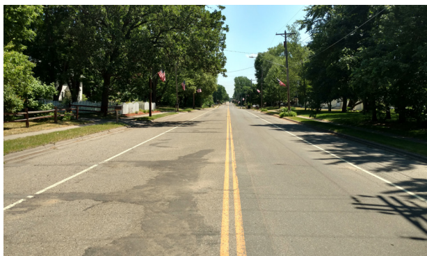
Just West of Fenwick Avenue Looking East
