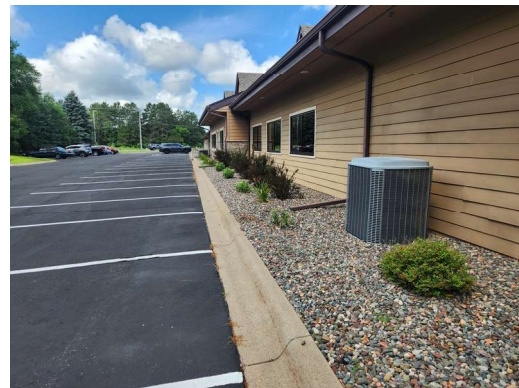
6. South elevation from the southeast
