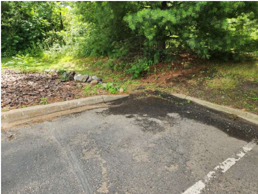
9. Southeast parking lot corner
