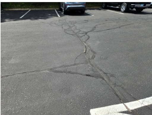
11. Asphalt temp repairs
