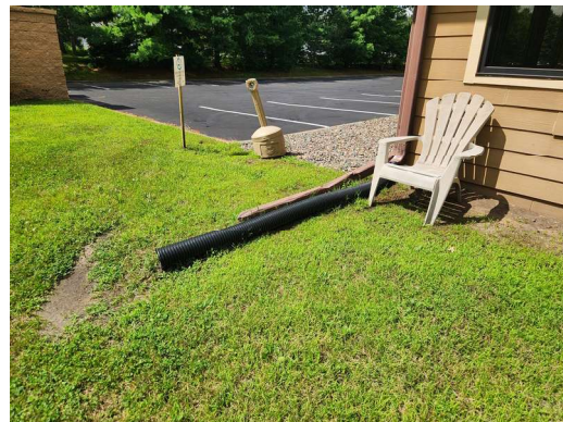
24. Typical roof drainage
