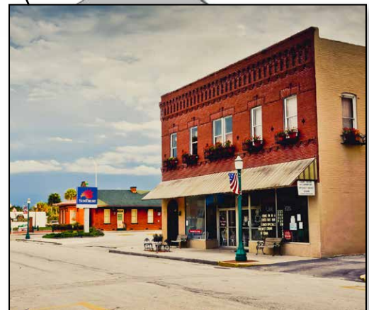
New mixed-use building
