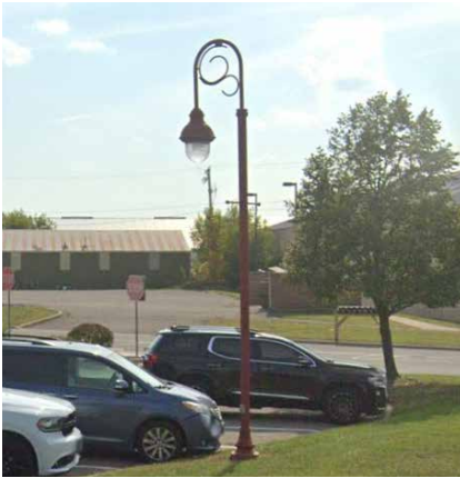
Existing light poles in highway commercial area.
