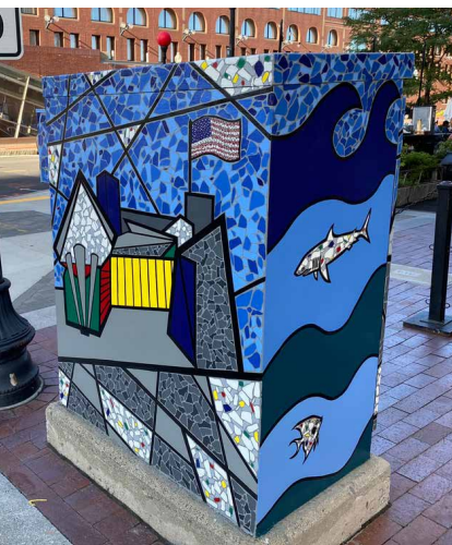
Example: Painted electrical box.
