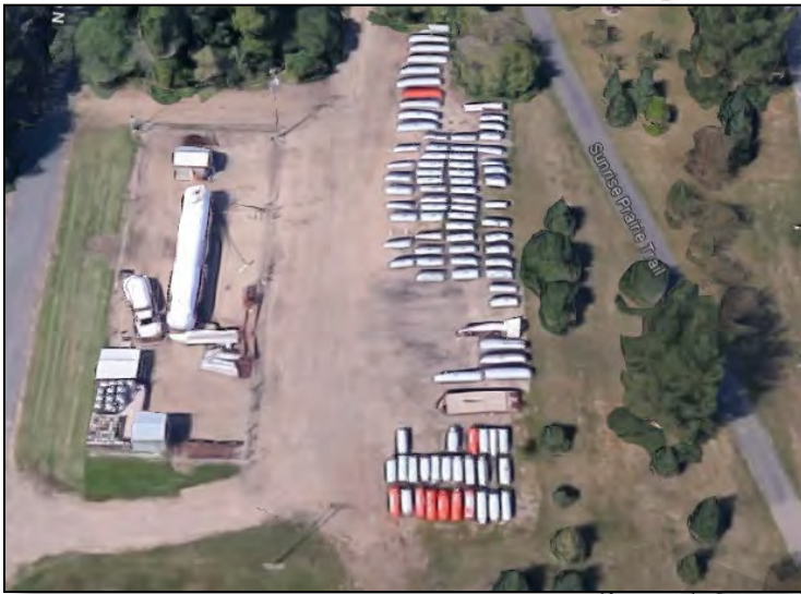
Gas tank storage, adjacent to Railroad Park
