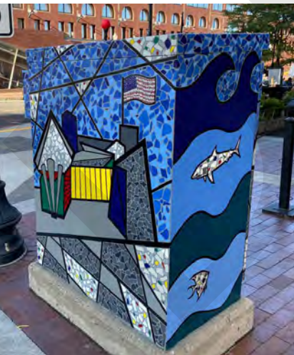
Example: Painted electrical box.
