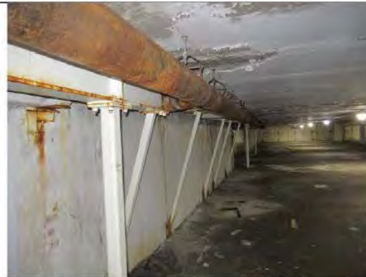
Photo 34: 7250 Parking ramp structural steel shoring
