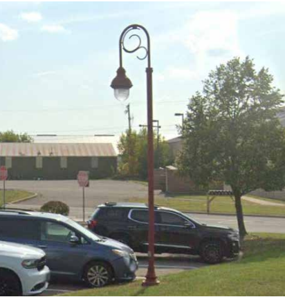
Existing light poles in highway commercial area.
