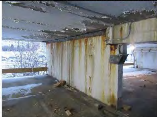
Photo 35: 7250 Parking ramp deterioration at bearing wall and steel angles and plates added to support deck above
