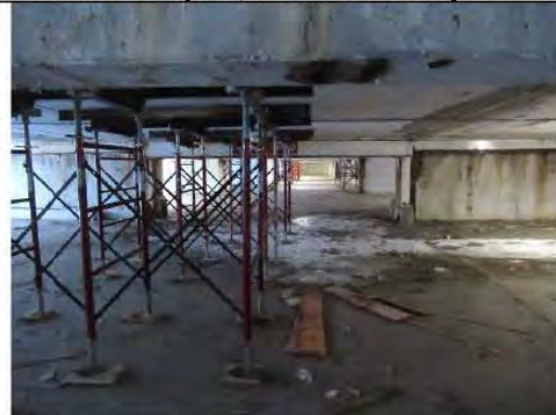
Photo 36: 7250 Parking ramp temporary shoring
