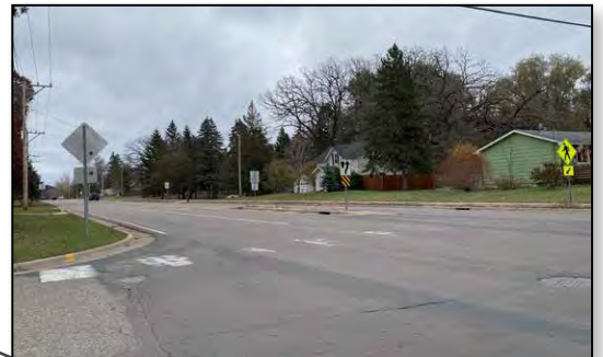
Wyoming Trl/Fenwick intersection, looking southeast
