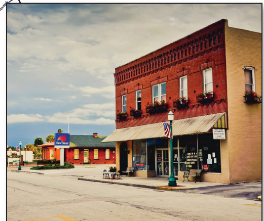
New mixed-use building
