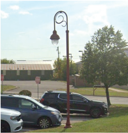
Existing light poles in highway commercial area.
