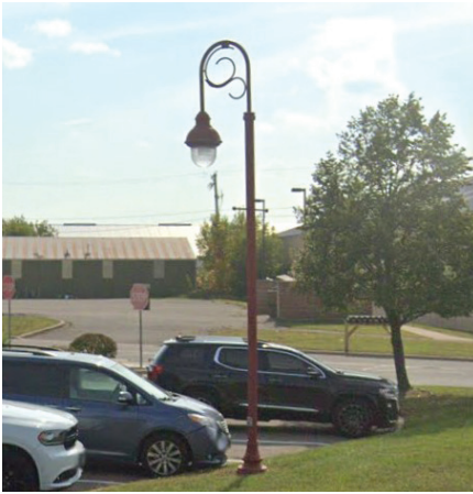
Existing light poles in highway commercial area.
