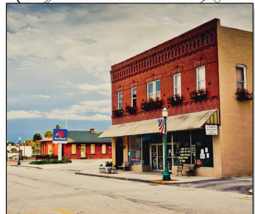
New mixed-use building
